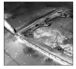
\* If using the frame on the outside of the duct, a continuous liquid tight weld is required. Care should be taken to not warp the frame when welding.
