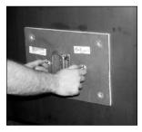
5. Tighten wingnuts and bolts with washers in corner holes.
