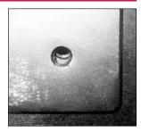
4a. NOT CENTERED If you can see the wall of the duct through any of the corner holes, then it is not centered.
