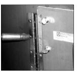
7. Install the bolts with washers. For hinged door, position hinge on duct wall and plug weld.
