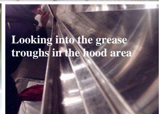
Looking up from the hood into the grease duct, partially inspecting the horizontal plenum area
