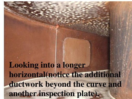
Looking into a horizontal above A hood drop-(notice the additional ductwork beyond the curve).
