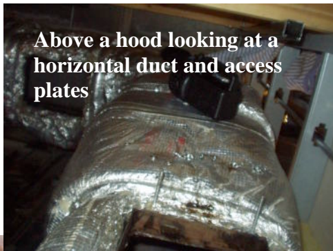
Looking inside a typical horizontal plenum for a "T" system above the hood.
